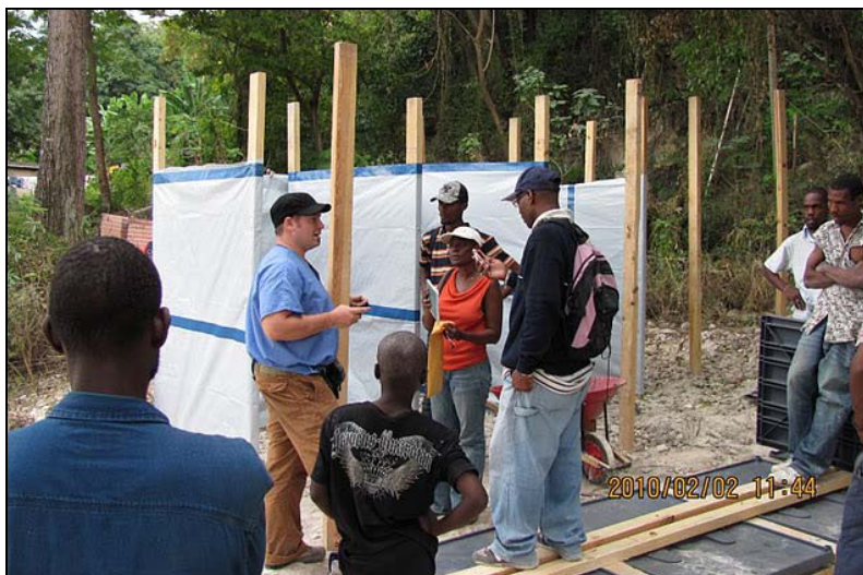
Above: A successful trench latrine program involves camp residents in every step of the planning and training processes. Although a significant amount went into digging the latrines, an equal amount of effort went into logistics and communication with camp leaders. Photo courtesy Ryan Sinclair.
